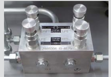
Load regulation block: Cylinders & motors
